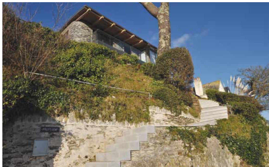
There are a total of 82 steps from the house down to the concealed parking area below the property. Due to the nature of the site, 1,600 tonnes of rock had to be excavated before construction work could begin
